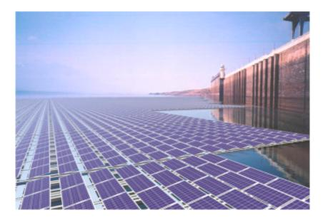
Fig. 1 A floating solar photovoltaic system (Cazzaniga 2018).
